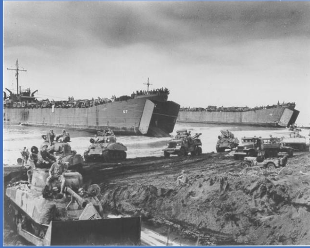
Unloading at Noemfoor
